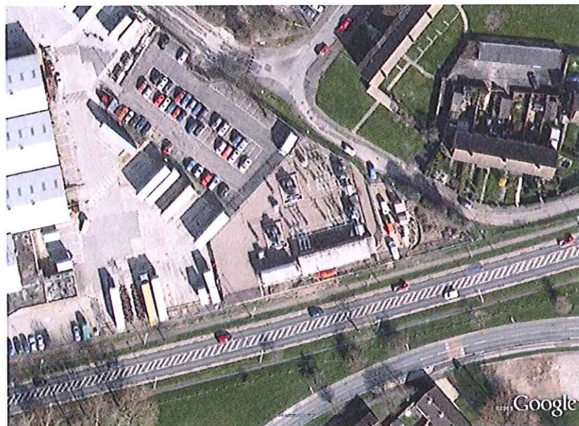
Figure 3: Tuffley 33/11kV Substation
