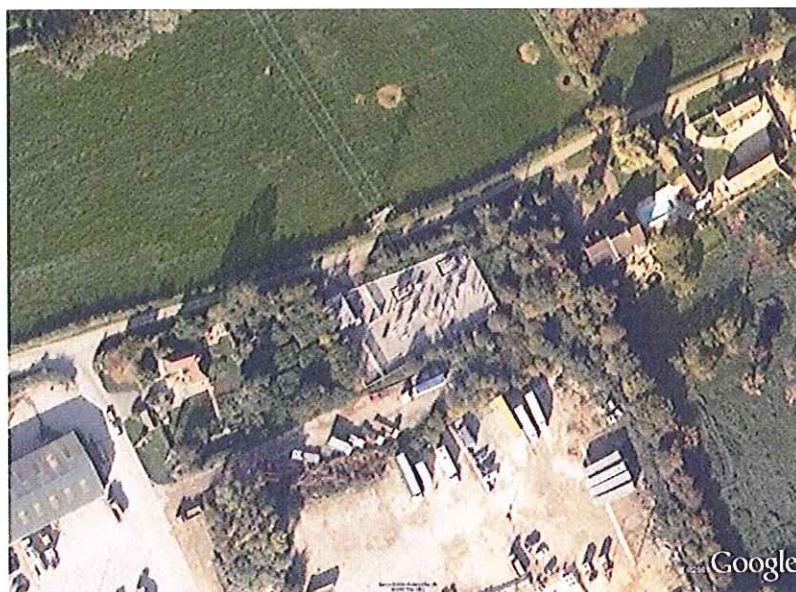
Figure 4: Netherhills 33/11kV Substation
