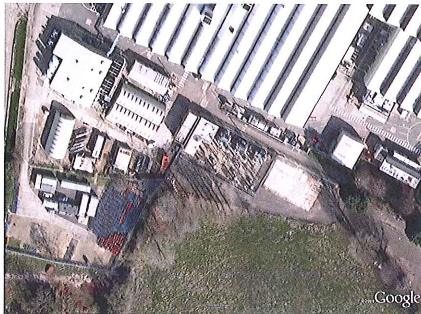
Figure 6: Brockworth 33/11kV Substation
