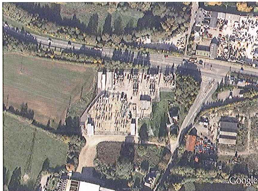
Figure 5: Ryeford 132/33/11kV Substation
