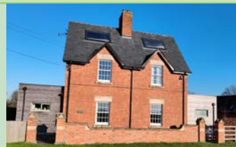
Retrofitted house on Standish Lane
