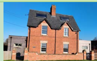
Retrofitted house on Standish Lane
